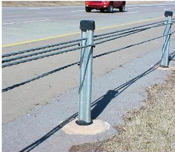
**Figure 1.1** Brifen High tension Wire Rope Safety Fence (TL-4)
